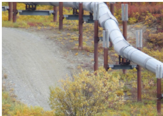
Photo of Alaska Pipeline.
